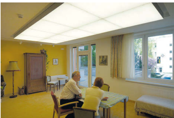
Fig. 4-4. Luminous ceiling in the living room area. The colour temperature and illuminance can be modified as described.
