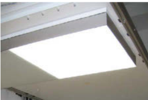
Fig. 4-2. One element of the light fields in the common area with the "CIELOS special" luminaire
