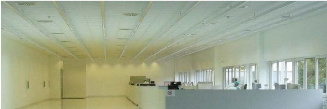
Production bay shortly after installation of the lighting in 2005. The bay has not been fully furnished yet, and the sections of the bay are deliberately operated using two different lighting conditions for demonstration purposes, in order to illustrate the varying colour temperatures.
