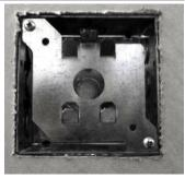
Raise fixture up and toward wall onte 3 dual hook of hanger bracket (on wall box) to hang fixture fixture. Connect corresponding wires (not shown).
