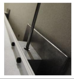
Proper installation places fixture canopy tight to wall with no gaps.
