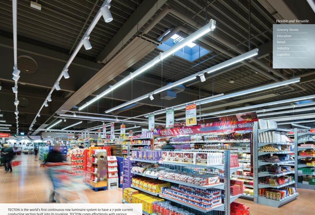
TECTON is the world's first continuous-row luminaire system to have a 7-pole current conducting section built into its trunking. TECTON copes effortlessly with various lighting requirements – at the time it is installed and whenever there are changes. The trunking system forms the functional backbone and then it is simply a matter of replacing or adding luminaire elements, light sources or optics as required.
