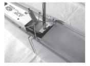
Reinsert the lens into the second fixture by pressing starting at one end and working your way to the other end, being sure that all LEDs are covered.
